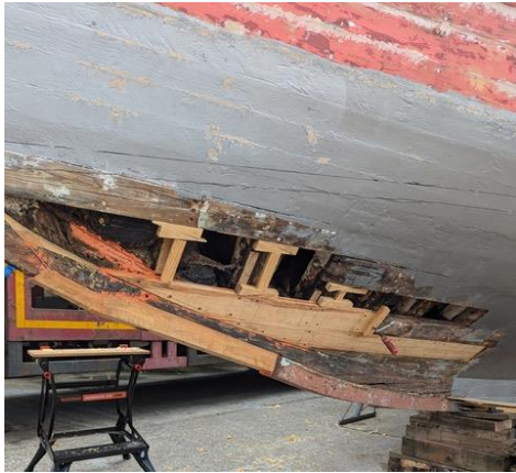
Photo showing planking repairs in progress
